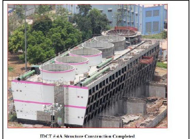
TDCT #4A Structure Construction Completed
